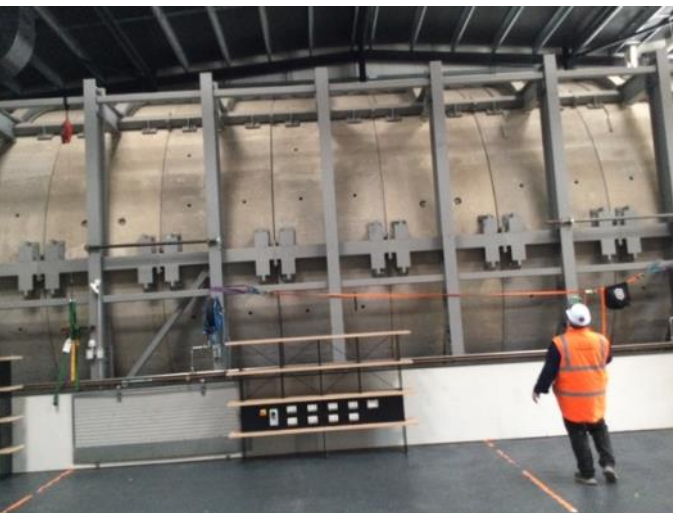
Outside view of the segmented rail tunnel
